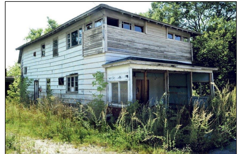
Abandoned house in Winslow
