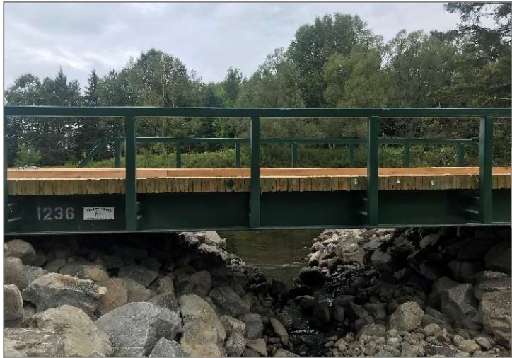
New bridge to enhance stream and riparian area function at Bigelow Unit, BPL Western Region
